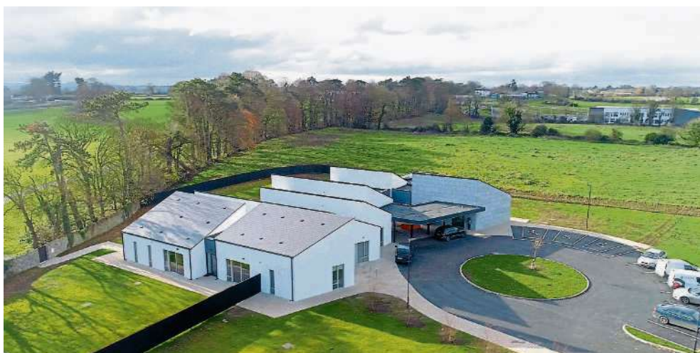
An aerial shot of the completed respite centre in Mungret
