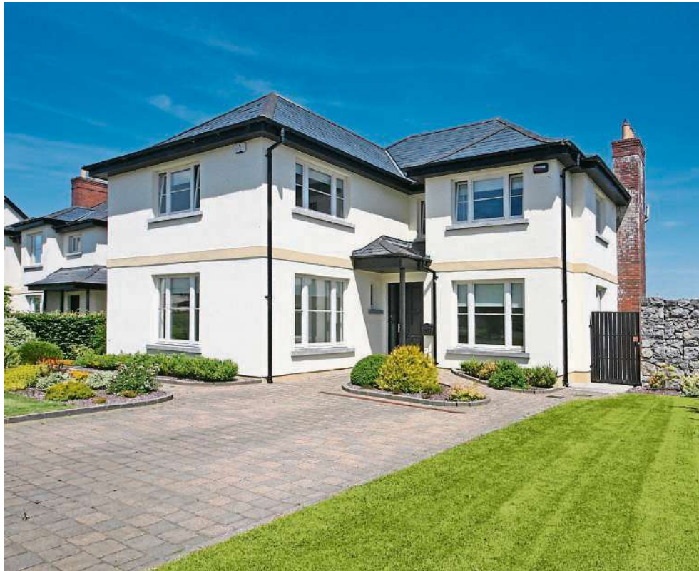
This large, well-appointed family home boasts a fantastic location in Adare Above left: the living room has a feature marble fireplace and polished solid wood flooring
