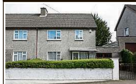
16 St. James Court, Ennis Road
