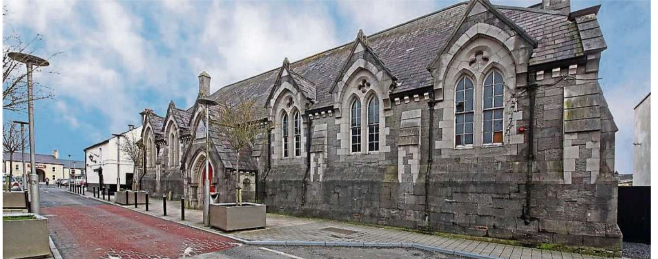
The former St Joseph's School building in Kilcock is being converted into a shop and restaurant. PICTURE: GOOGLE MAPS
